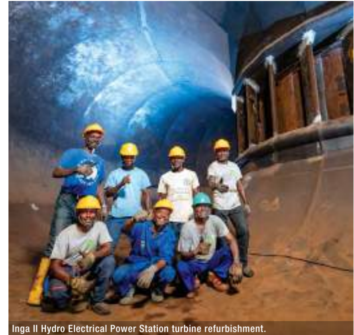
Inga II Hydro Electrical Power Station turbine refurbishment.
