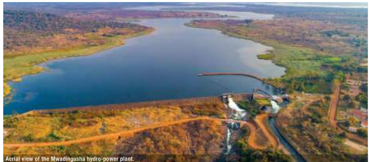
Aerial view of the Mwadingusha hydro-power plant.
