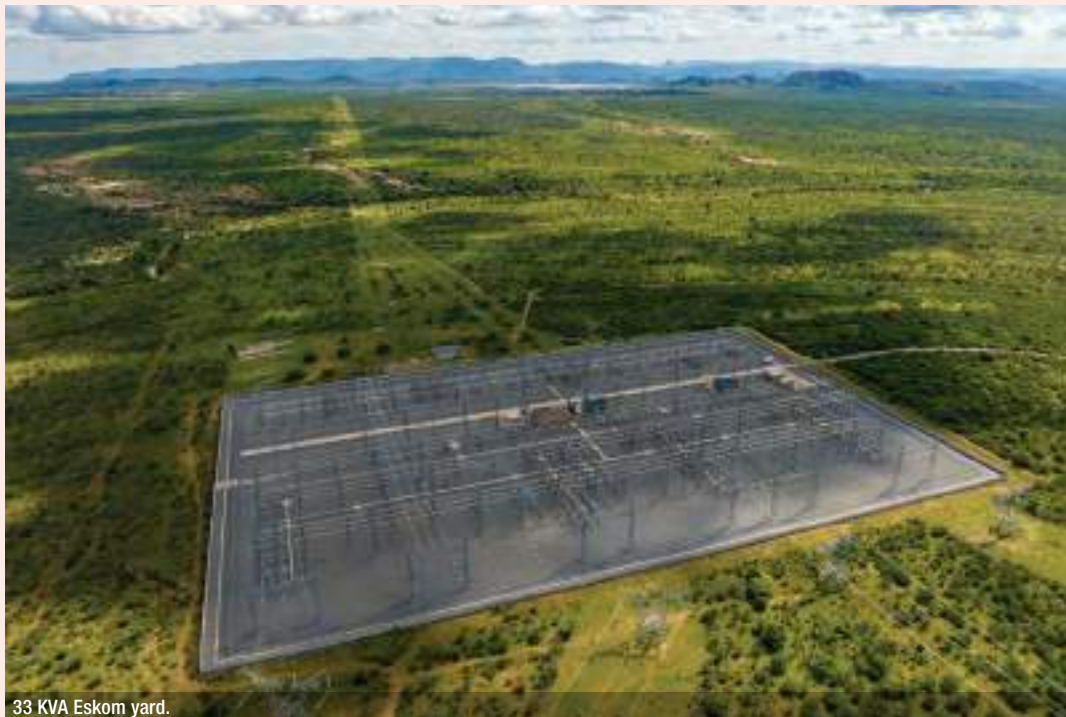
33 KVA Eskom yard.
